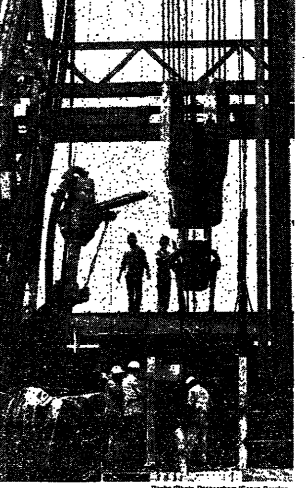
Drilling rig is mounted on a barge in the river. The Nigerian Government is now rigidly controlling oil wealth.
